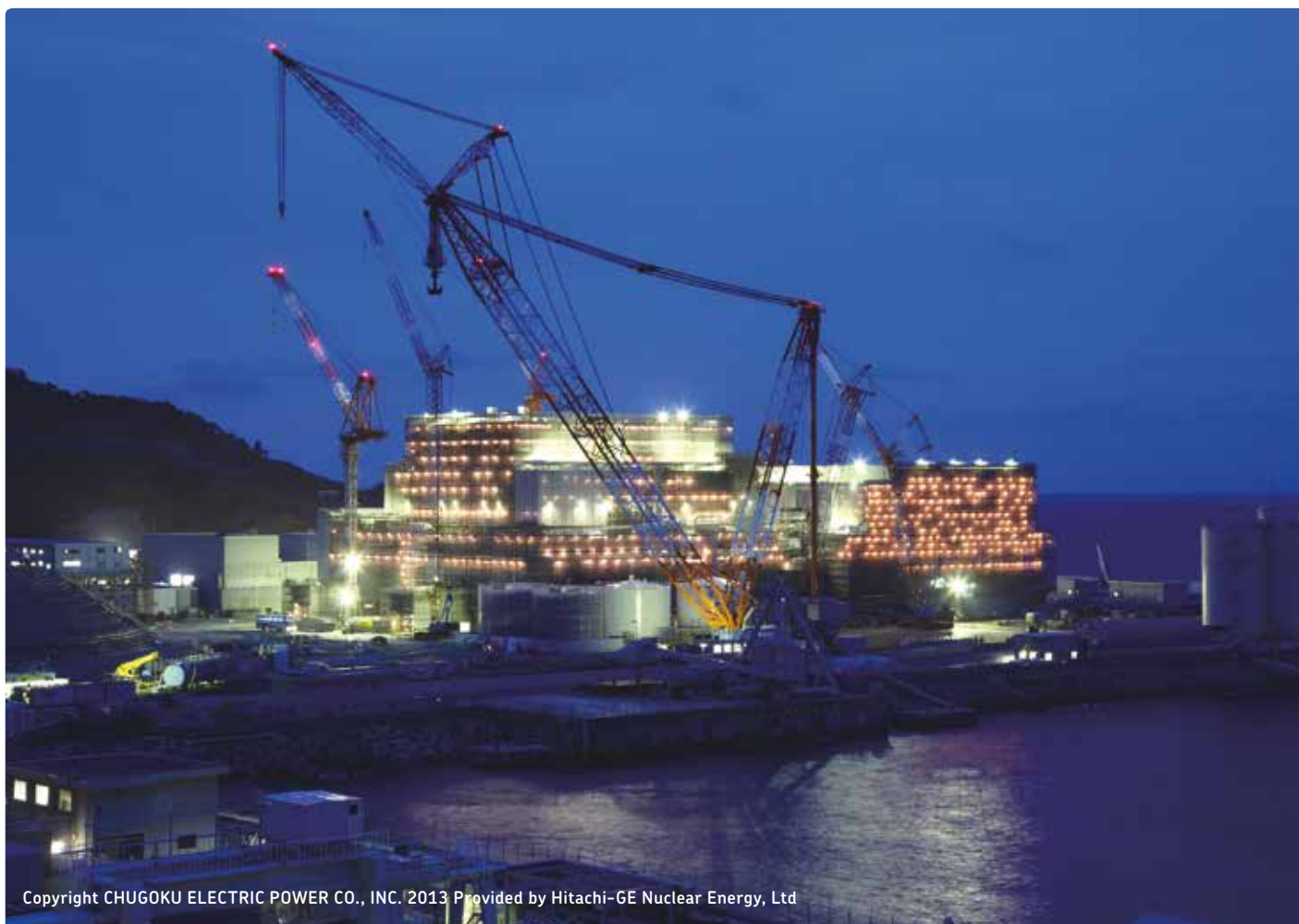
Figure 2: Construction of ABWR building at Shimane 3 in Japan
